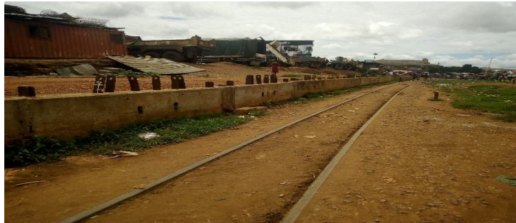
Plate 3.14: Status of the existing rail infrastructure
