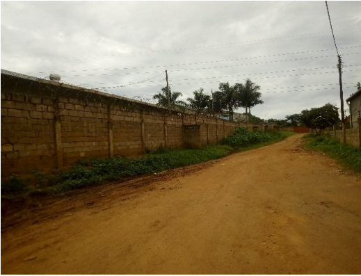
Plate 3.7: Roads without side drains
