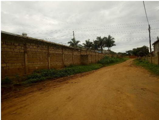
Plate 3.7: Roads without side drains
